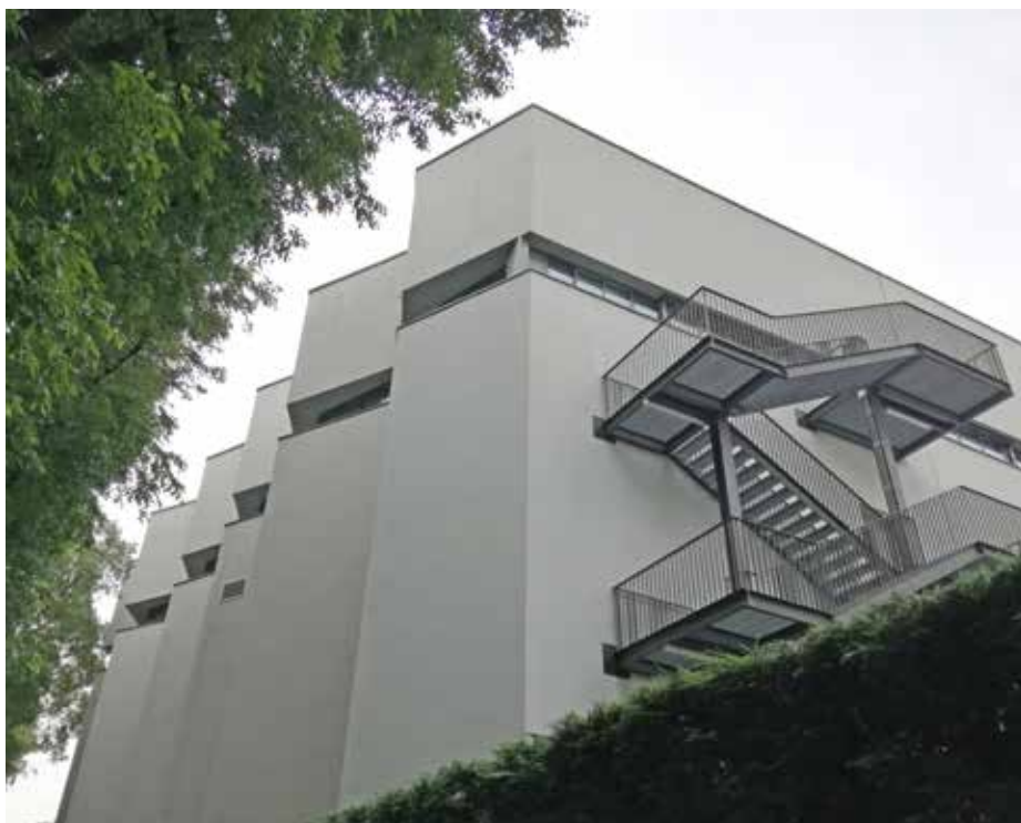
18. Armani Silos. Exterior view of the East and North facades and Interior view of the central empty volume (photo by S. Landi)
