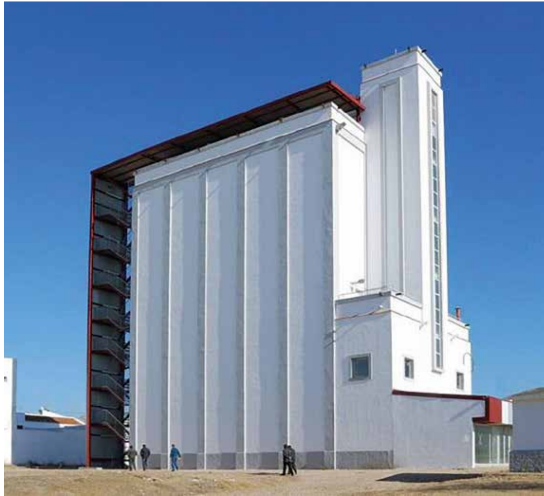
15. Silo in Fuente de Andalucia after conservation (photo by Fábrica de Arquitectura archive)
